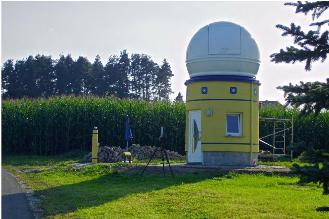
Figure 3, The Sternwarte Rotheul Observatory by Henry Bolgehn, in Germany, the cupola is a 3 metre ScopeDome with tower design based on drawings by Narkowicz-Pala. (*Henry Bolgehn 2011*).
